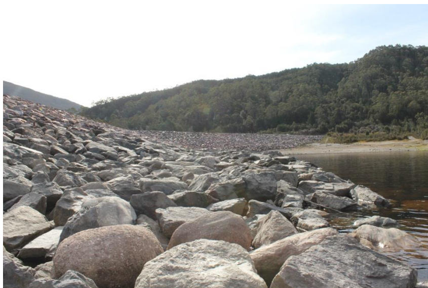
Figure 3. The Darwin Dam (image courtesy of Danielle Fairfield).
